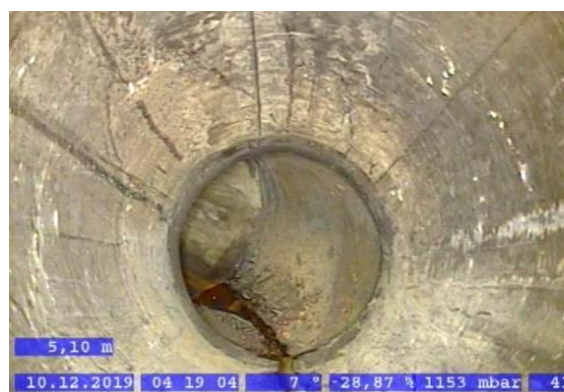
Figure 4. Host pipe 45° bend
