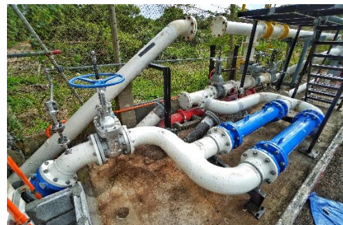
Figure 8. Tie-in during construction
