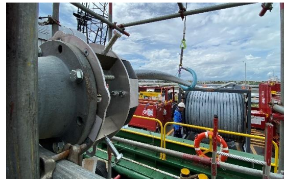
Figure 13. Liner installation phase
