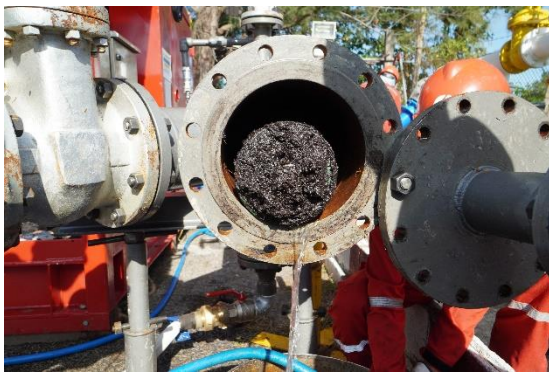
Figure 9. Cleaning pig at the pig receiver
